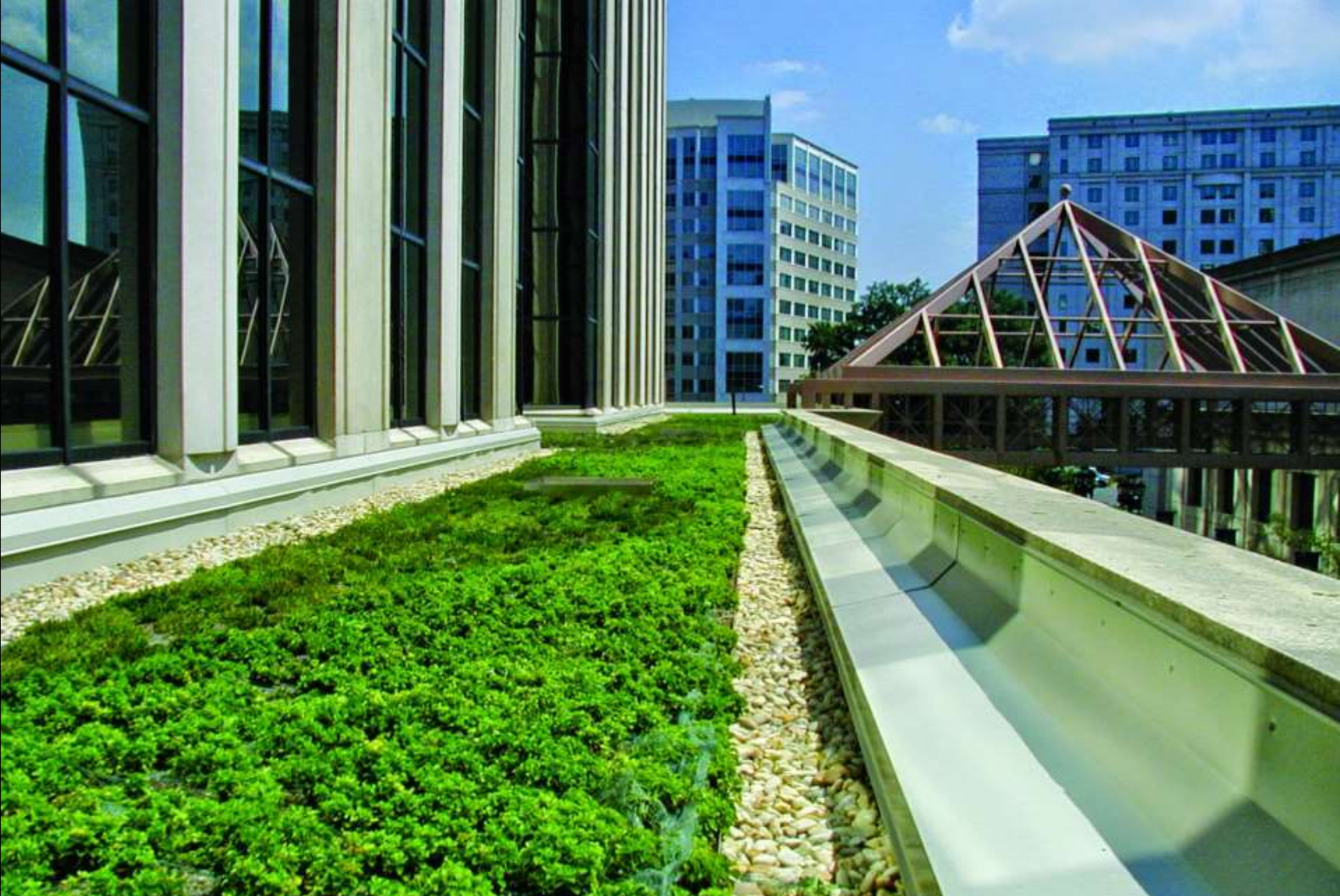
Arlington County Government – Green Roof
